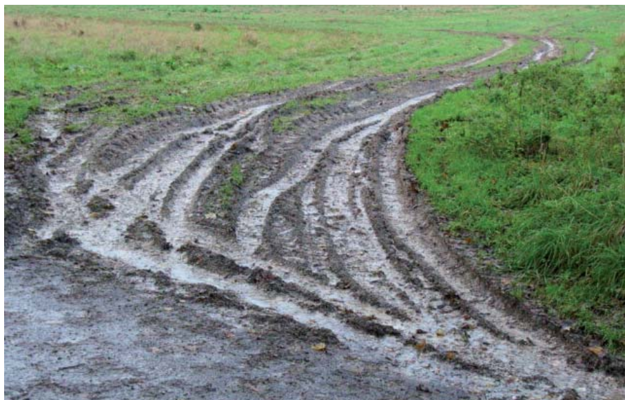
Ruts caused by too much traffic during wet weather and now acting as a channel for run-off and a source of erosion.
